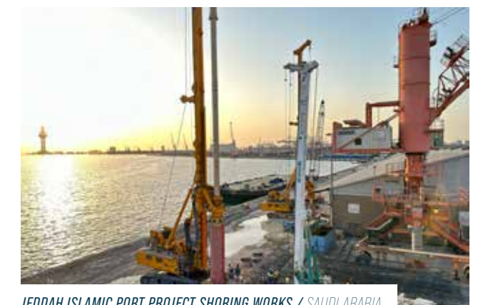
JEDDAH ISLAMIC PORT PROJECT SHORING WORKS / SAUDI ARABIA
